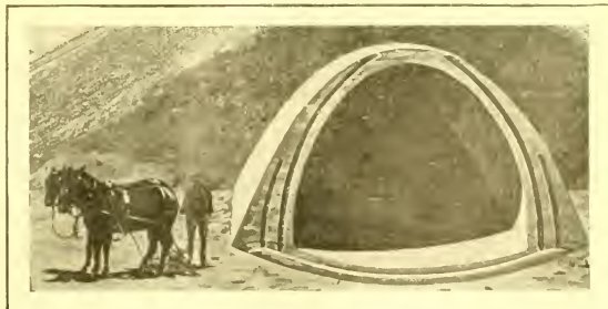
A section of the tunnel which carries water from the Ashokan Dam to New York. Compare the size of the entrance with that of the team of horses.
